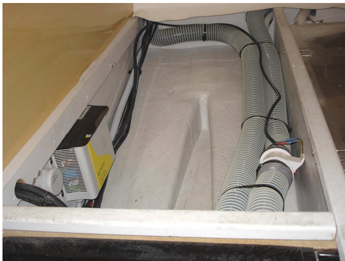
Battery charger in port cabin beneath bunk
